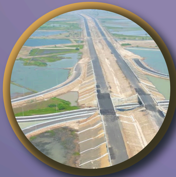
250m WIDE & 6 LANE AHMEDABAD DHOLERA EXPRESSWAY
