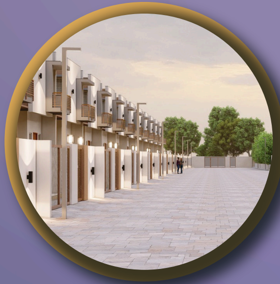
INTERNAL ROAD STREET LIGHTS
