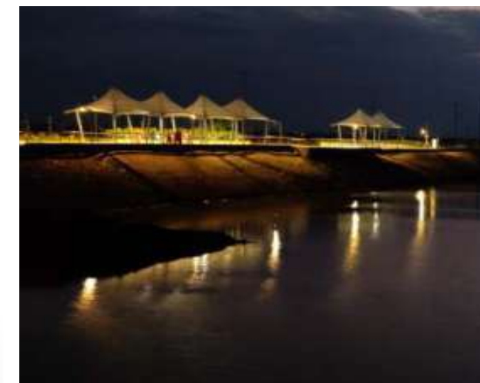
Canal & Canal Front 6.5 km Long Canal for Storm Water Management, Canal Front to be used as Recreation Zone
