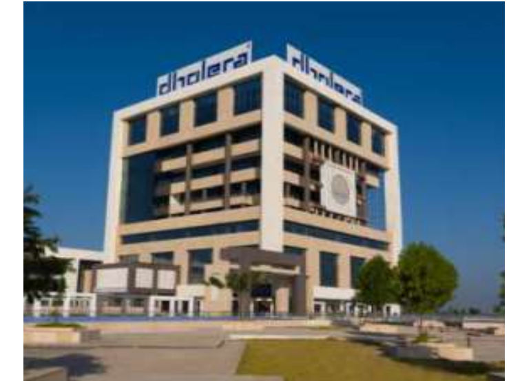
ABCD Building Administrative Building with City Integrated Operation Center
