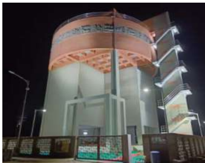
Water Supply & Storage Infrastructure 2 Master Balancing Reservoirs and 9 Elevated Service Reservoirs
