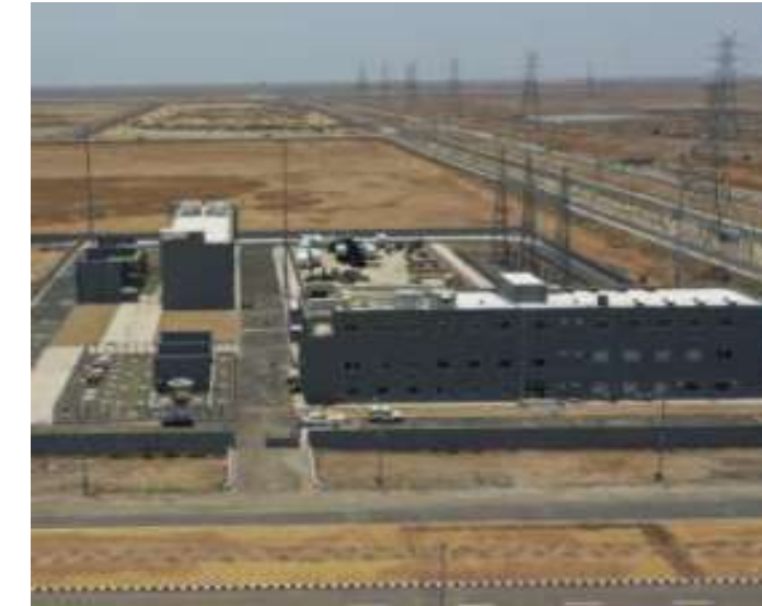
Power Substations 2 Substations (33/66 kv and 220 kv GIS) by Torrent Power
