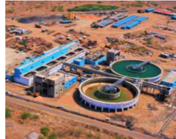
Water Treatment Plant 50 MLD Commissioned, expandable up to 150 MLD
