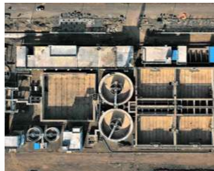
Common Effluent Treatment Plant 20 MLD Commissioned, expandable up to 60 MLD
